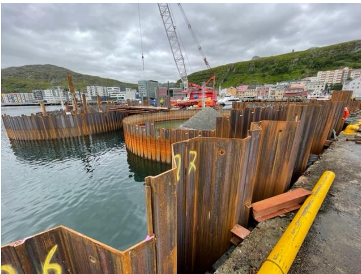
Cellespunddeponi for forurensede mudringsmasser.
